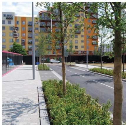
Integrated rain gardens & parallel parking bays
