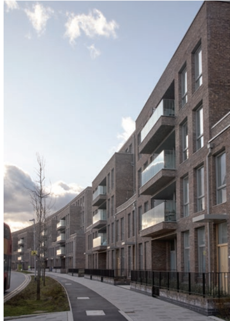
New housing at Barking Riverside
