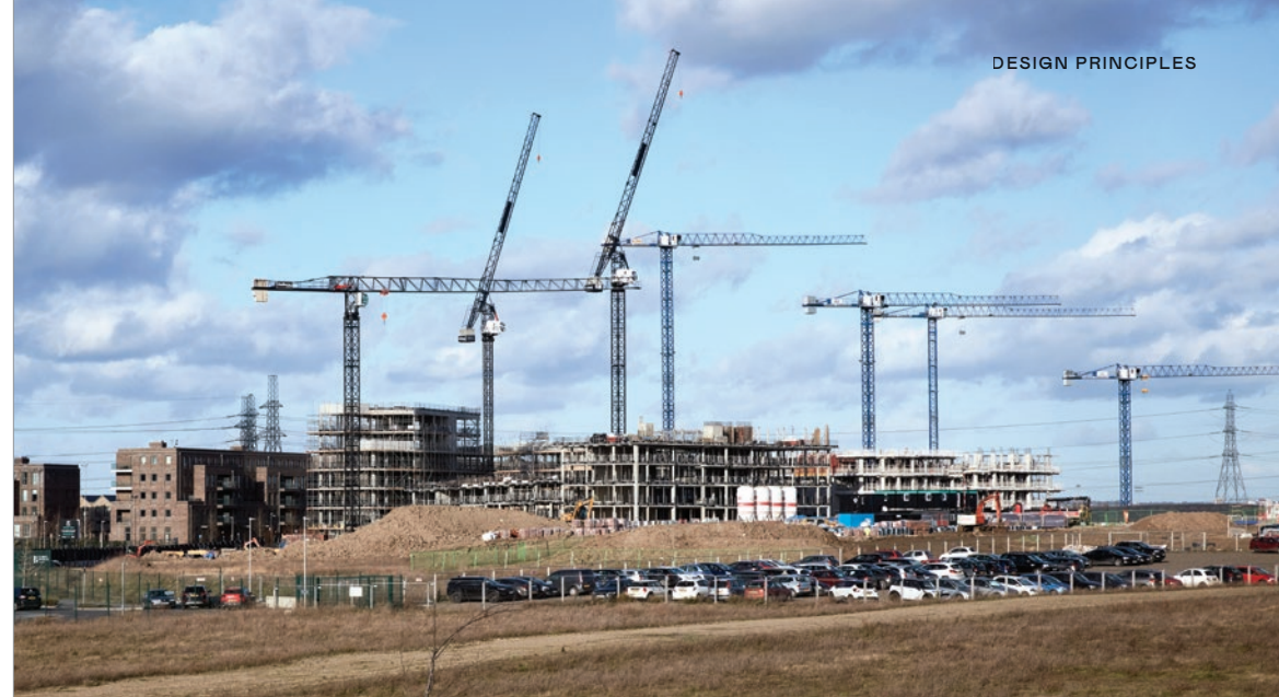
Regeneration in progress at Barking Riverside
